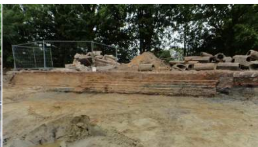
Foto 6: gemetselde fundering Z87
